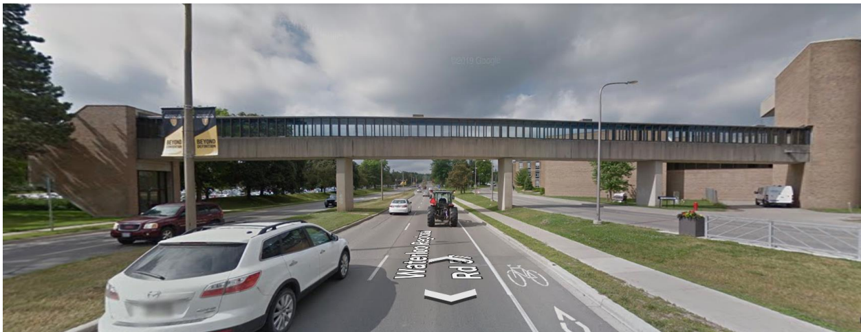
Figure 1.1 Google Maps street view of the existing bridge
